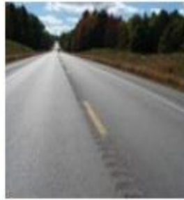
2-Lane Roads 80–90km/h (Milled rumble strips)
